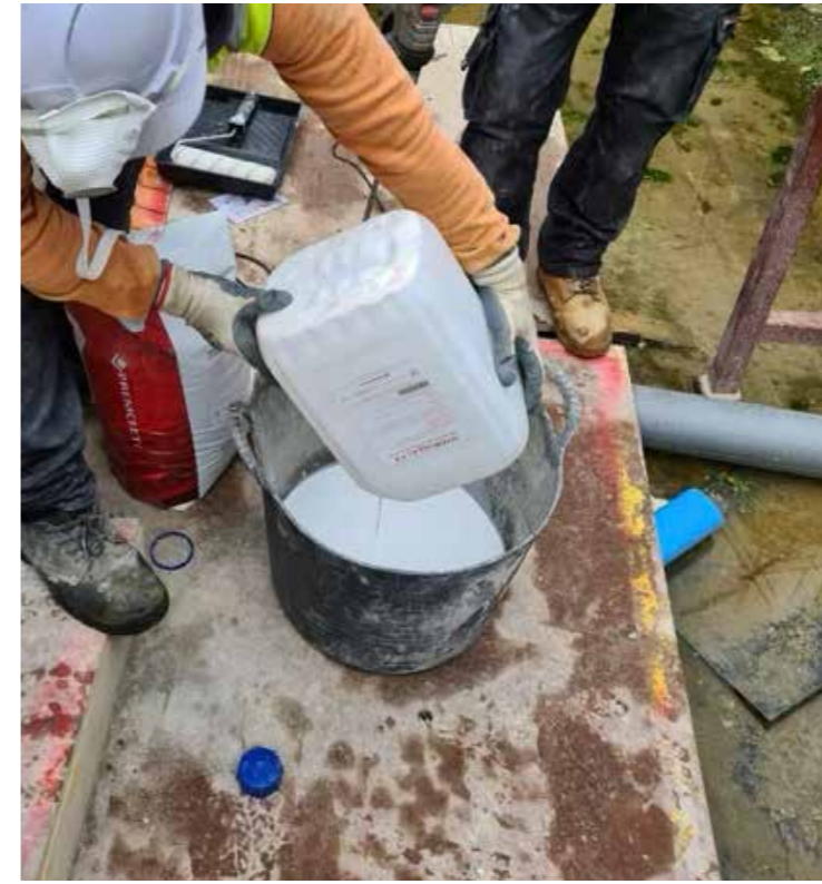
Hydroseal FX should be mixed with mechanical whisk using 1 tub of liquid to 1 bag of powder and mixed for at least 5 minutes to ensure the correct consistency. No part mixing is acceptable.
