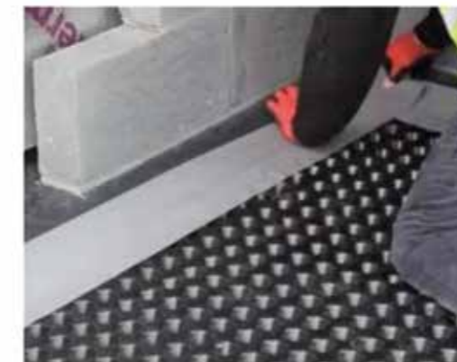
Tape the Hydroprufe DPC to the Hydroflow HP20 using Hydroflow Corner Tape.
