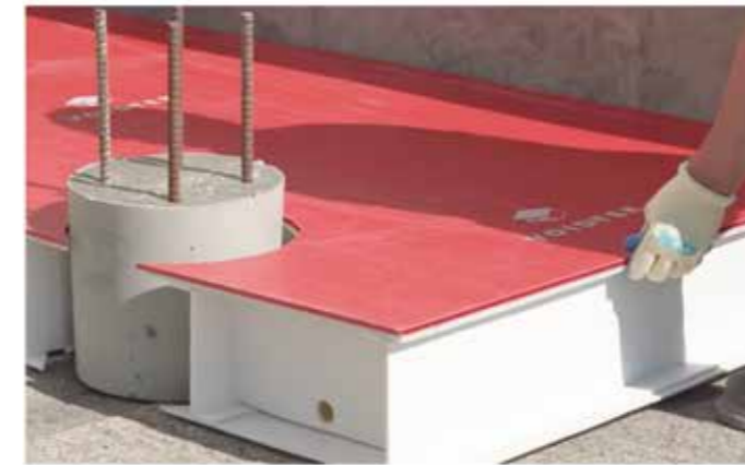
Place in position, lowering over the pile.
