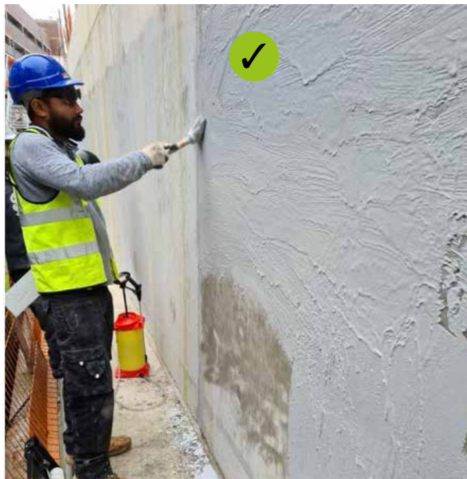
Hydroseal FX can be applied by brush or trowel to a minimum thickness of 2mm. On vertical surfaces the coating will need to be applied in two 1mm layers to ensure a 2mm layer.
