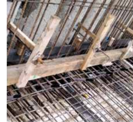
Cemflex VB to be secured between starter bars.
