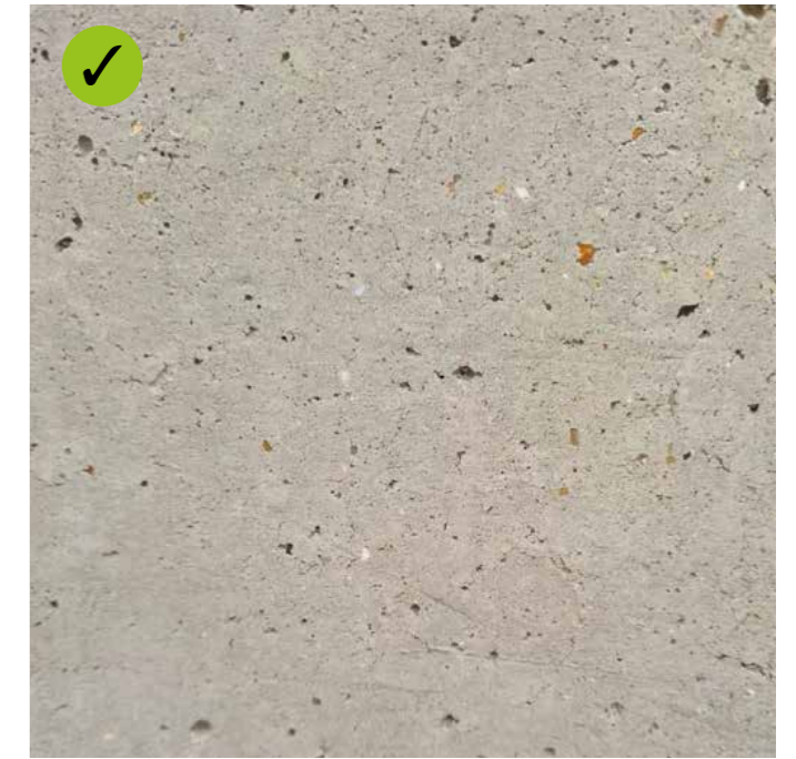
Example of suitably prepared wall. Note that the surface is rough and aggregate exposed.
