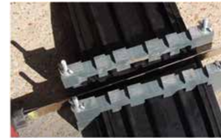
Position the hot knife between the ends of the Hydrobar and slide the second Hydrobar into the hot knife.
