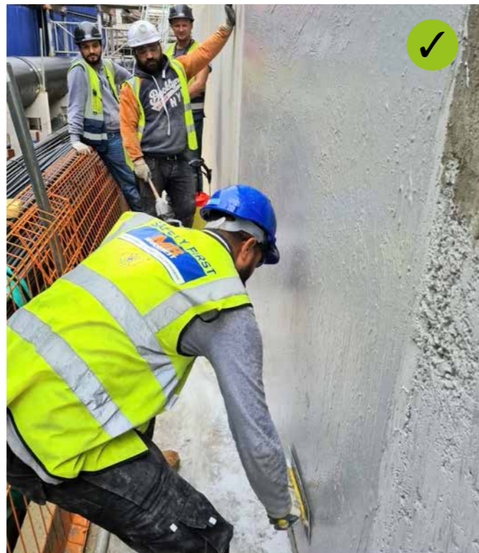
Hydroseal FX being applied by trowel.
