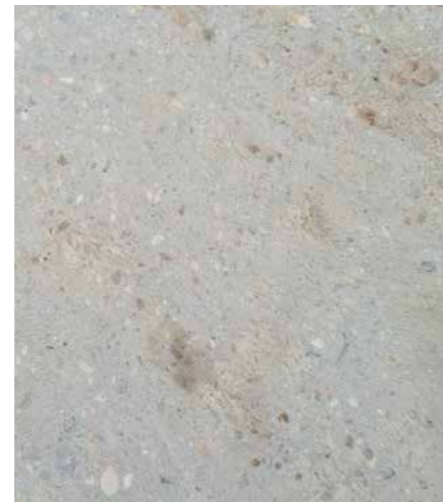
Example of correctly prepared substrate.
