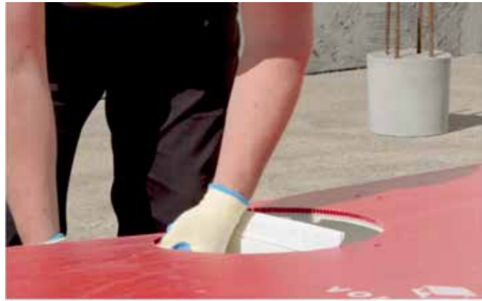
If there is a structural fin revealed below, cut it with a stanley knife and also remove the interlocking flap.
