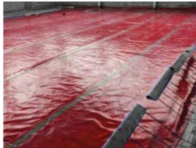
Membrane prior to protection board installation.
