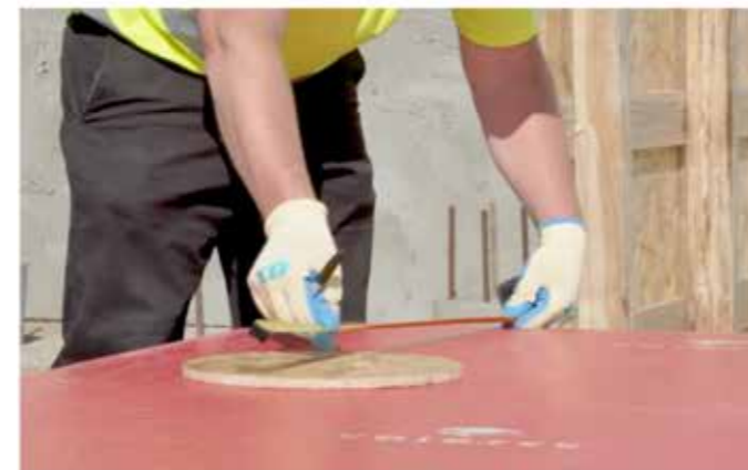
Create a template for the pilehead or pile cap and place in position on the Void-Tek panel.
