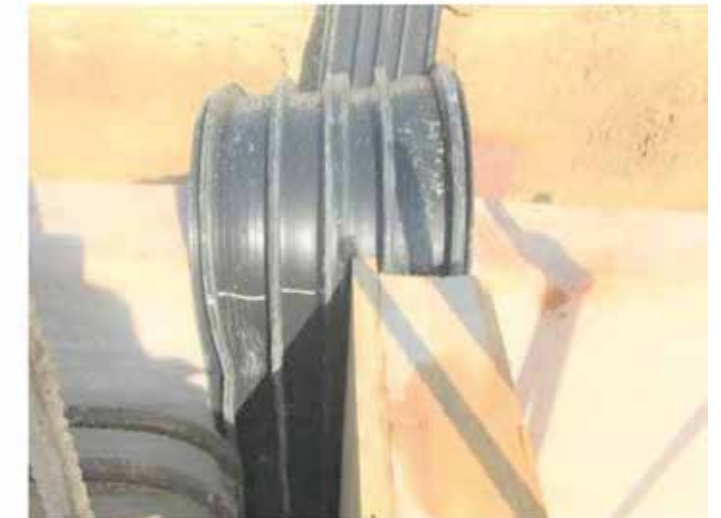
Exafoam board should be Installed against the shutter and then pour the concrete.
