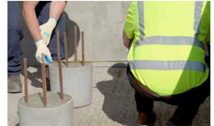
Accurately measure the pile cap diameter.
