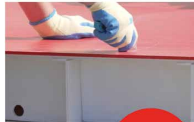
Cut the top of the board with a stanley knife and expose the area below.
