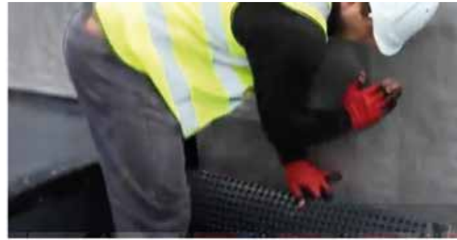
Adhere Hydroflow HM8 drainage membrane to the vertical surface once self adhesive membrane has been installed, using high adhesion double-sided tape.
