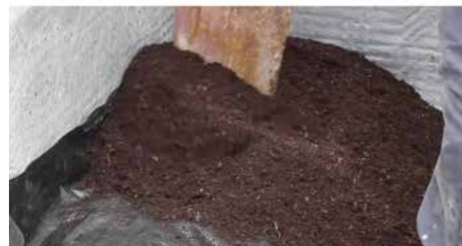
With the land drain protected, backfill with soil or other substrate as required.
