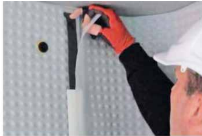
Remove release paper and firmly push adjacent membrane to bond together.
