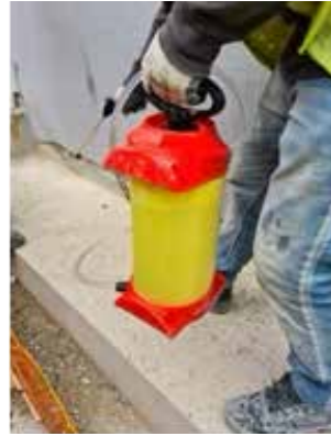
Saturate the substrate with water using a suitable sprayer.
