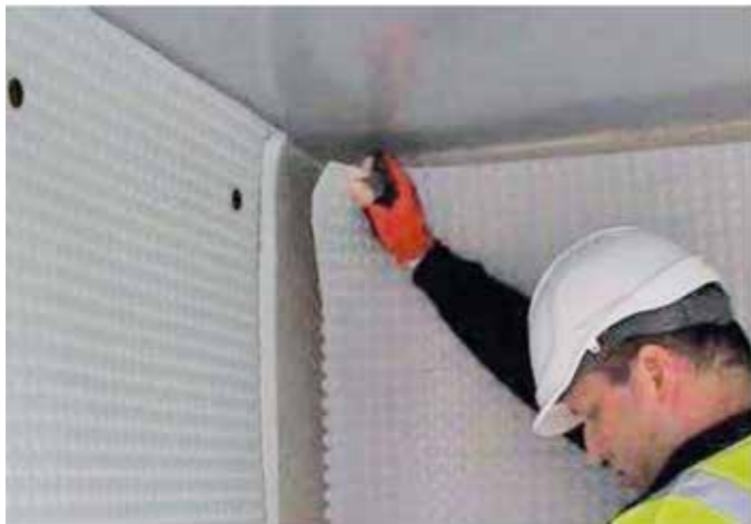
Ensure laps are placed 200mm from the corner.
