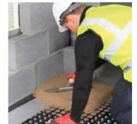
Once complete, Hydroflow HP20 is ready to receive floor screed.
