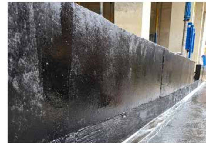
For slab edge detailing, follow the same procedures as outlined above for substrate preparation, primer application, membrane application, and protection with Protection Board 600, taking particular care to achieve neat, continuous coverage.
