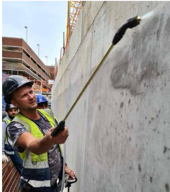
Surface prior to preparation. This substrate would not be suitable to receive a coating of Hydroseal FX.
