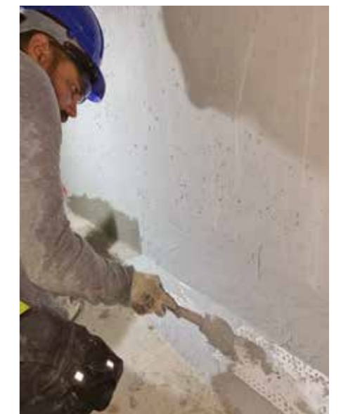
Hydroband 2000 is to be applied over any areas susceptible to cracking. Apply a 2mm layer of Hydroseal FX and embed the Hydroband 2000 into the layer. Then apply a second 1mm layer of Hydroseal FX over the top of the Hydroband 2000.
