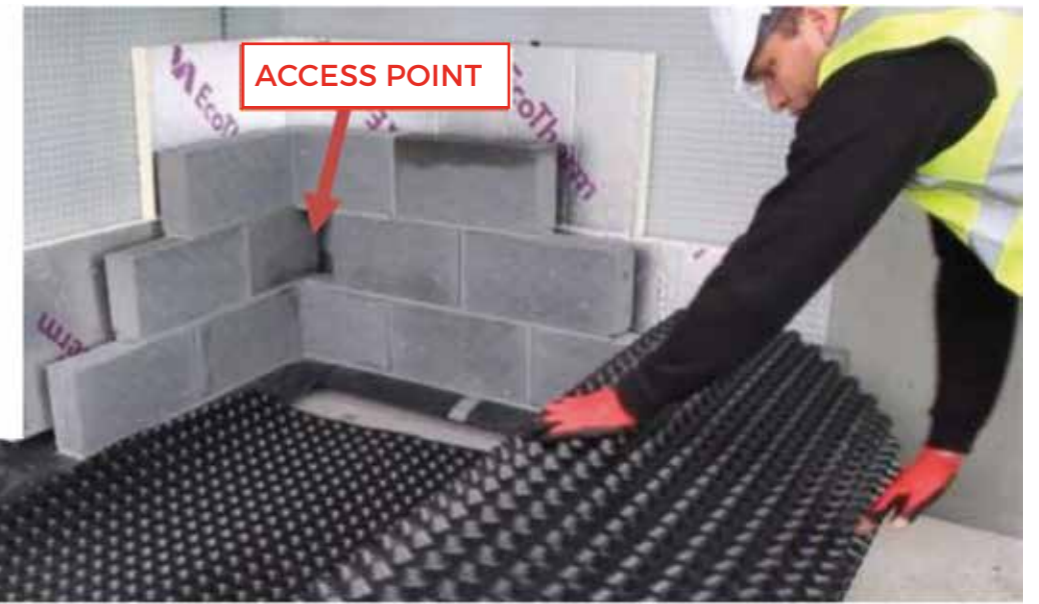
Roll Hydroflow HP20 out on the floor with studs facing down.
