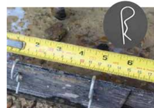
Overlap waterbar by minimum 150mm ensuring plates are held tightly together. Two Cemflex clips should be used to secure each lap.
