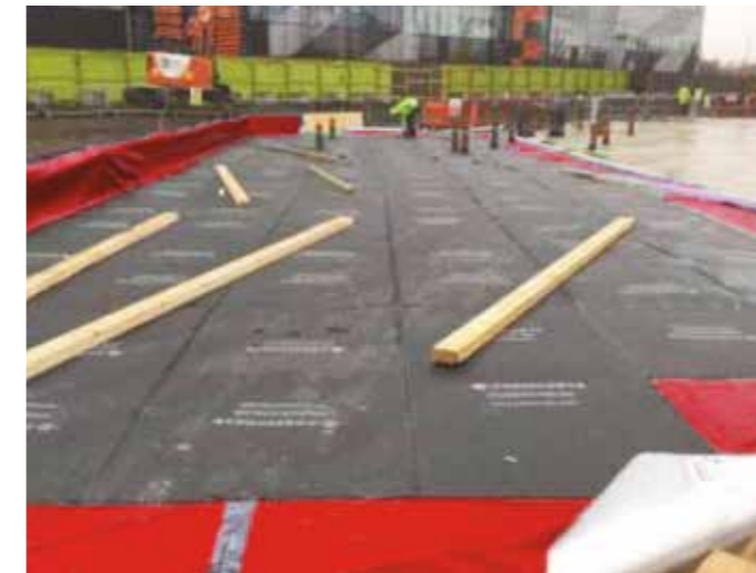
Protection board 300 to be installed to protect membrane from puncture. Spacer blocks can then be installed.
