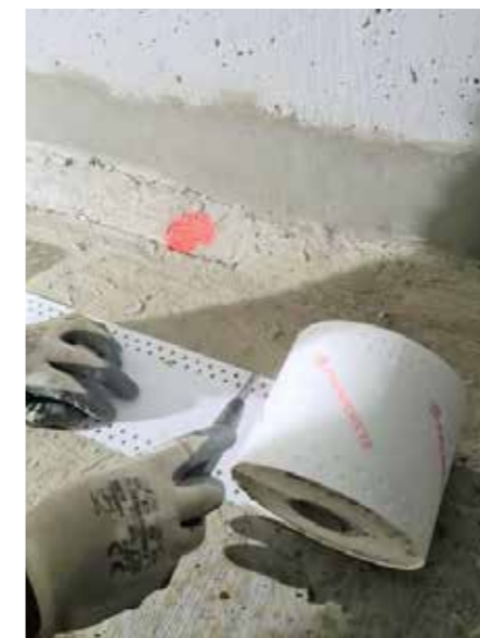
Hydroband 2000 is to be applied over any areas susceptible to cracking. Apply a 2mm layer of Hydroseal FX and embed the Hydroband 2000 into the layer. Then apply a second 1mm layer of Hydroseal FX over the top of the Hydroband 2000.
