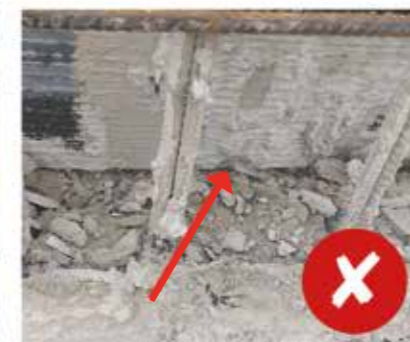
There must be no gap beneath the Cemflex VB after the first concrete pour.
