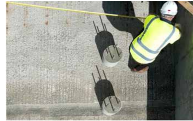
Set out and measure the area intended for Void-Tek positioning.
