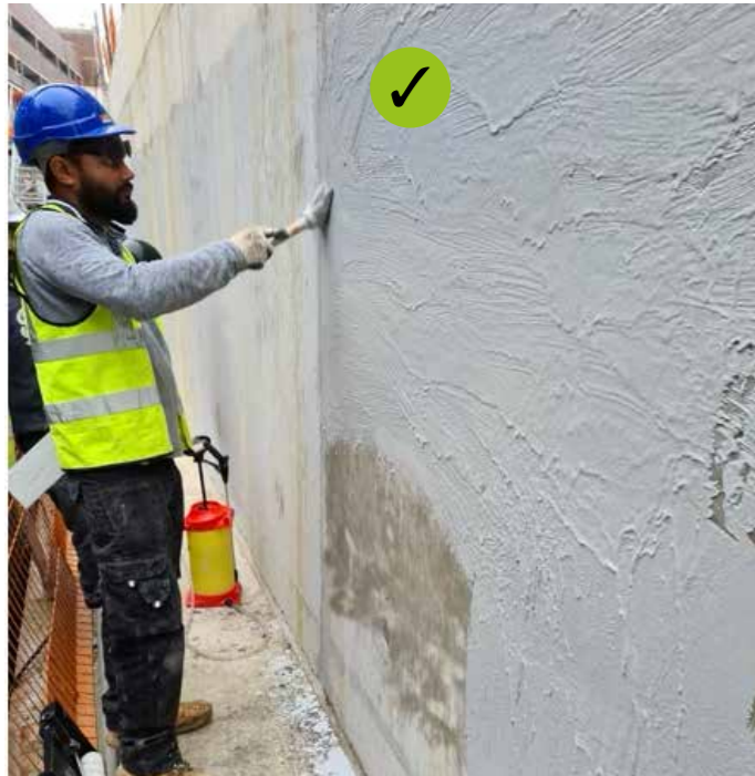
Hydroseal FX can be applied by brush or trowel to a minimum thickness of 2mm. On vertical surfaces the coating will need to be applied in two 1mm layers to ensure a 2mm layer.
