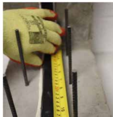
Nail waterbar at 300mm centres using Hydrostop retaining pins.
