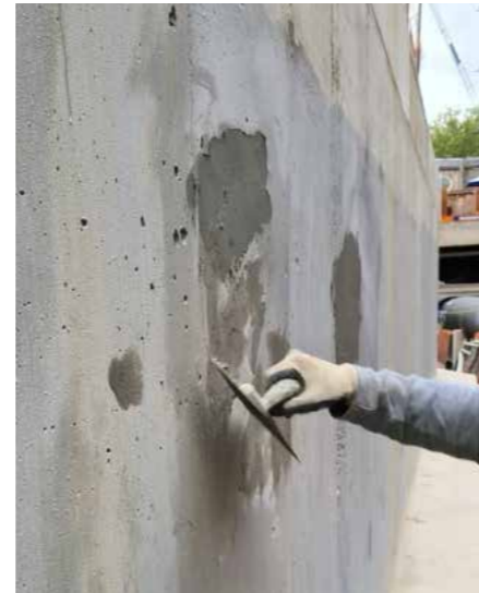
Teknolevel FS should then be used with a Trowel to fill in any pores on the face of the concrete.
