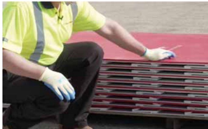
Place the Void-Tek flat panels near to installation area.
