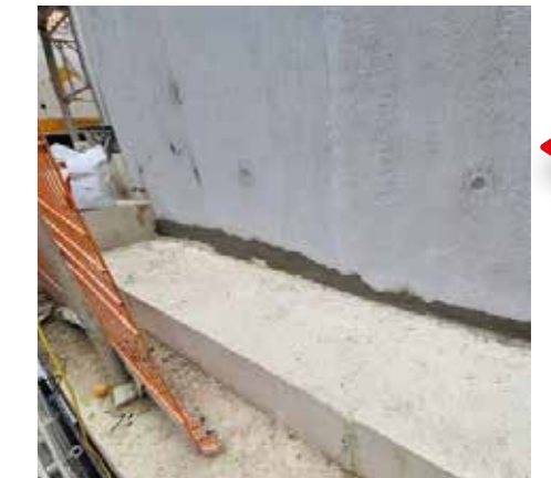
Mix the Teknocem HBR as per product instructions, and force into the gap with a gloved hand for initial contact coat, then build up flush with trowel.
