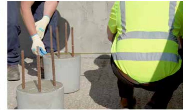
Accurately measure the pile cap diameter.
