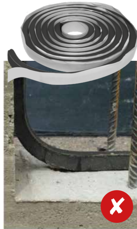
Butt joint internal corners to ensure there are no voids behind.
