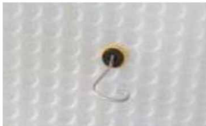
5mm diameter wall ties (Screw-in) can be used for brick/blockwork which are threaded into the pilot hole in the Hydroflow QS Plug.
