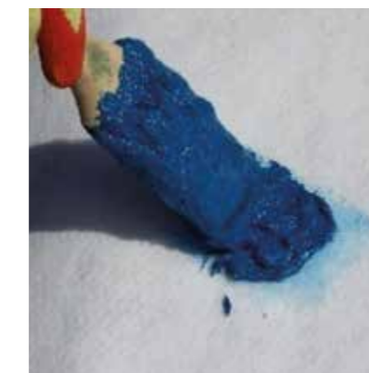
Where nails aren't fixed through the tape, overcoat the penetration with Twinseal Compound GR. These illustrations show CombiSeal Plus but the same principle applies for CombiSeal HD.
