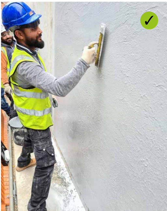
Hydroseal FX can be troweled to a smooth finish if required.
