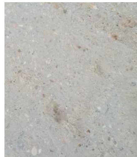
Example of correctly prepared substrate.
