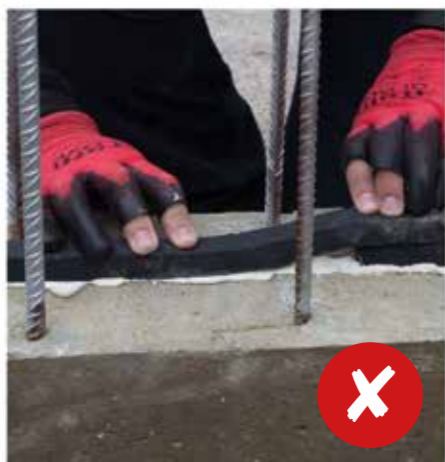
Joints in Hydrostop BR should be overlapped by a minimum of 50mm side-by-side. Install with a minimum of 75mm concrete cover to face of concrete.
