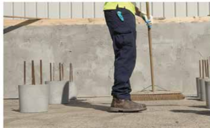
Sweep debris from concrete binding surface prior to laying Void-Tek panels.
