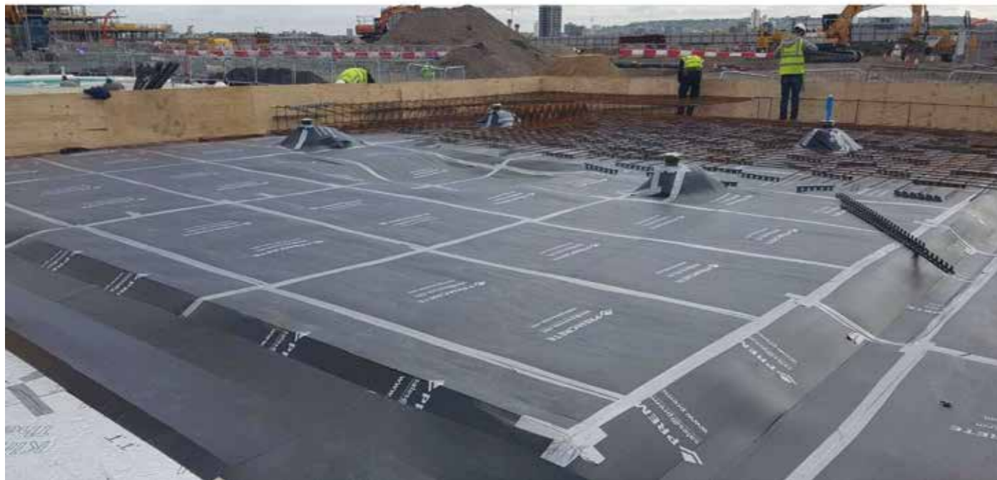
Protection Board 300 to be installed over the membrane to prevent damage from spacers and rebar.
