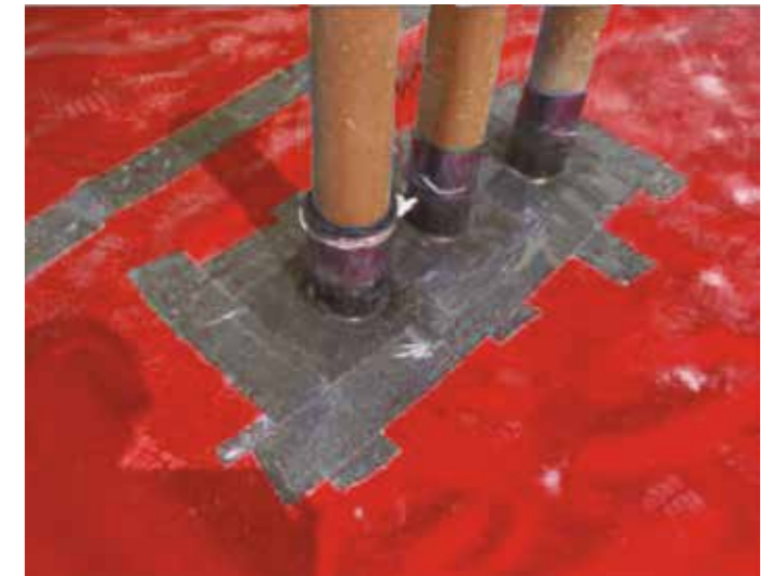
Seal using Hydroprufe Tophat to suit. Tape flanges to membrane using HRC Foil Girth Tape.
