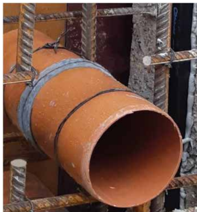
SMOOTH PIPE Apply Hydrostop WS10 directly to pipe using tying wire to secure. Overlap waterbar by 75mm side by side. Position to maintain a minimum of 75mm concrete cover.
