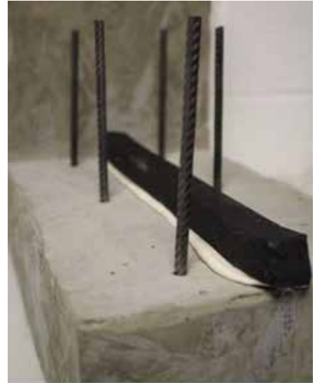
Firmly press the waterbar into Hydrostop WSM and ensure there are no voids below.
