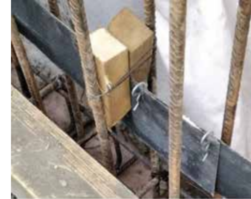
Cemflex VB should be pre-installed in kicker joint before concrete is cast. This can be hung with tying wire and timber blocks as pictured above, or Omega Holders can be supplied.
