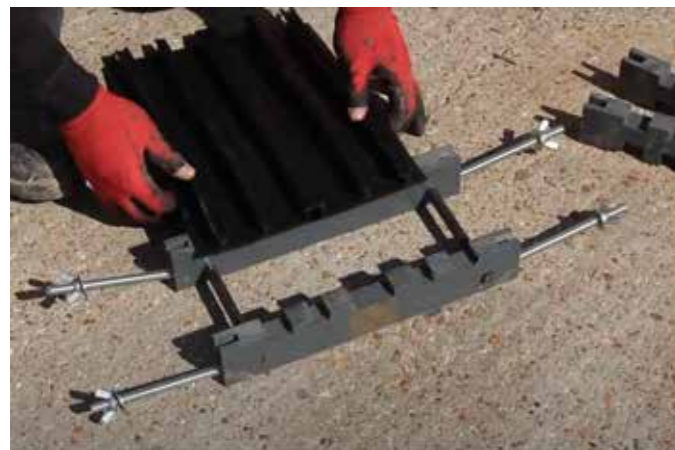
Lay Hydrobar onto the jointing jig.
