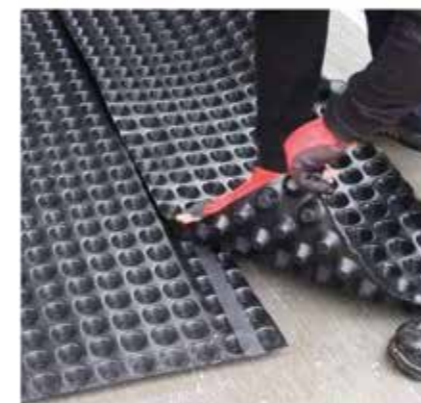
Ensure that Hydroflow HP20 is overlapped by a minimum of two studs and pushed firmly down to ensure the lap is sealed.
