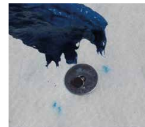
Where nails aren't fixed through the tape, overcoat the penetration with Twinseal Compound GR. These illustrations show CombiSeal Plus but the same principle applies for CombiSeal HD.
