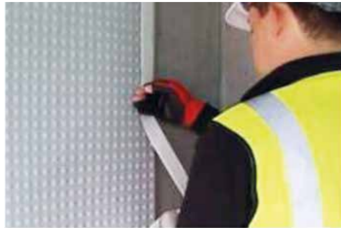
Laps should be sealed with Hydroflow Butyl Tape, 100mm from the membrane edge.
