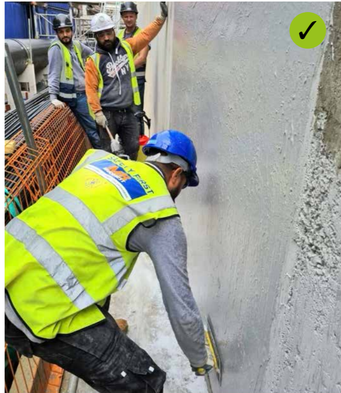
Hydroseal FX being applied by trowel.
