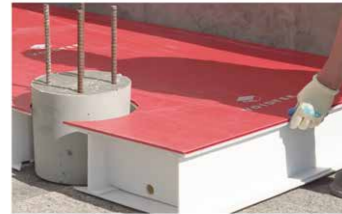
Place in position, lowering over the pile.
