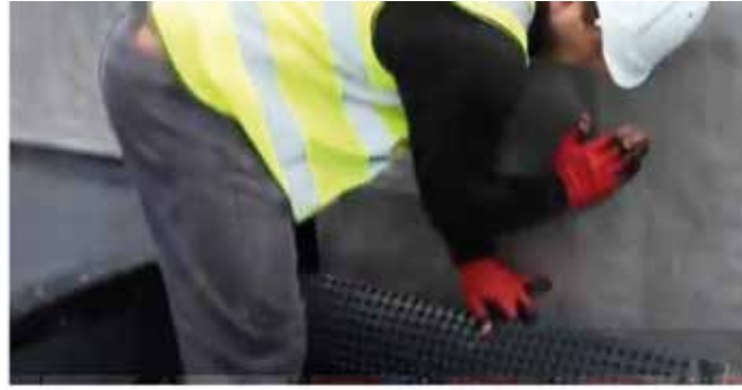
Adhere Hydroflow HM8 drainage membrane to the vertical surface once self adhesive membrane has been installed, using high adhesion double-sided tape.
