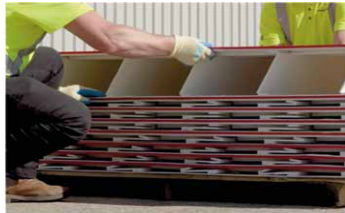
Lift top of Void-Tek panel to full height.
