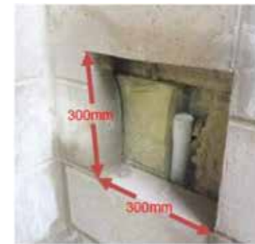
Recommended minimum access hatch size.
