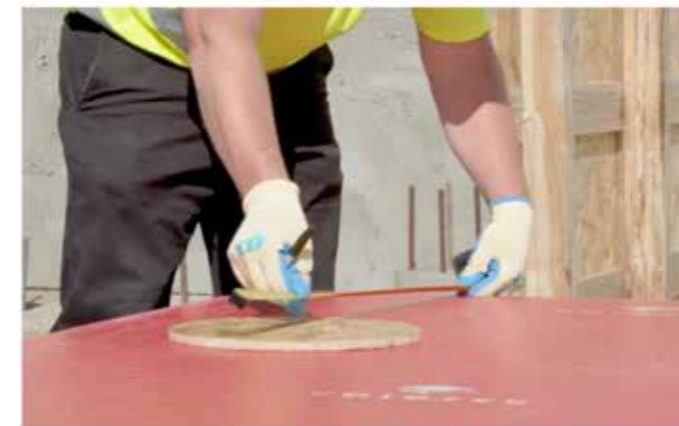
Create a template for the pilehead or pile cap and place in position on the Void-Tek panel.
