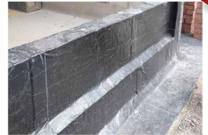
For best results, slab edge membranes should be applied as close as possible to the time of installing the brickwork façade or external cladding, as early installation without subsequent protection can leave the system vulnerable to site damage and compromise long-term performance.
