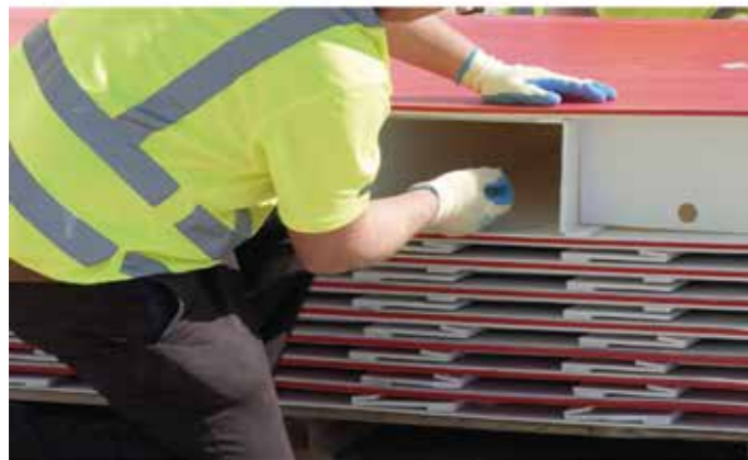
Pull down the interlocking flaps and lock into the slot provided.
