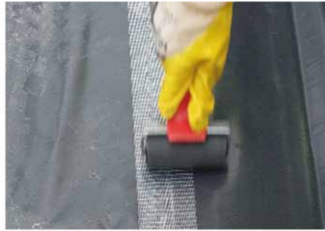
Minimum overlap should be 100mm. Laps to be sealed with 30mm HCR Butyl Tape within the lap and Girth Tape on the overlap. Laps should be rolled with a soft roller to ensure the tapes are fully bonded.
