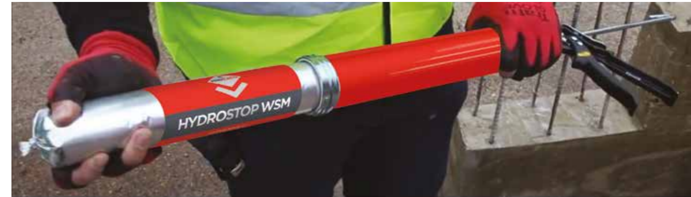
Insert Hydrostop WSM into applicator gun.
