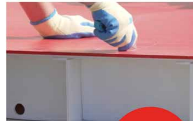
Cut the top of the board with a Stanley knife and expose the area below.
