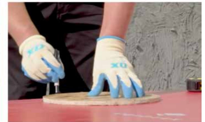
Once in position, mark up the areas to be cut with a permanent marker.
