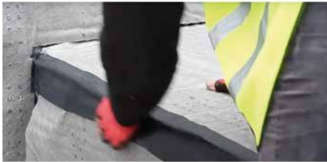
Seal all joints using high adhesion single sided tape.
