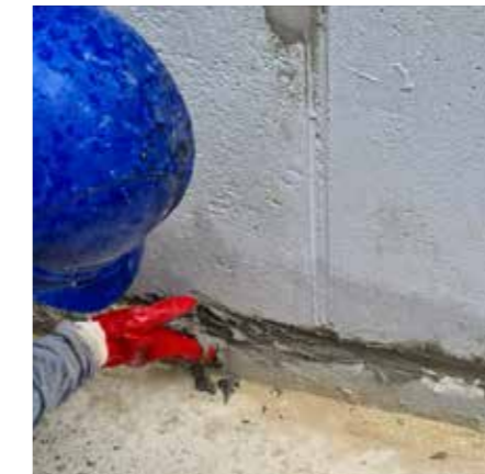
Mix the Teknocem HBR as per product instructions, and force into the gap with a gloved hand for initial contact coat, then build up flush with trowel.
