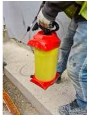
Saturate the substrate with water using a suitable sprayer.
