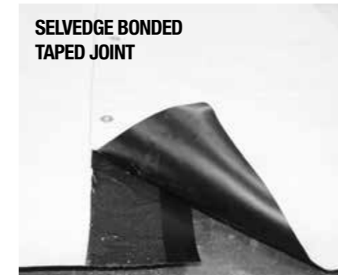
Remove white release paper from selvedge tape and butt joint the membrane ensuring a consistent seal along the lap.
