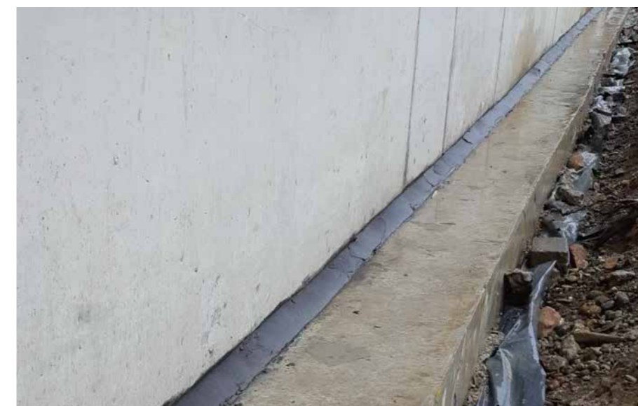
Mix the Teknocem HBR as per product instructions, and force into the gap with a gloved hand for initial contact coat, then build up flush with trowel.
