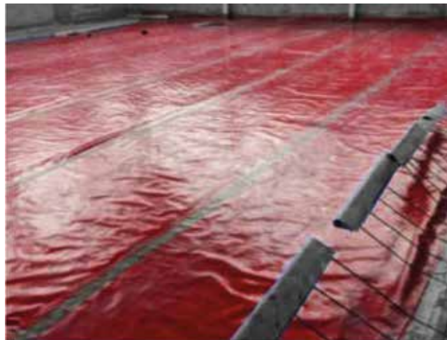
Membrane prior to protection board installation.
