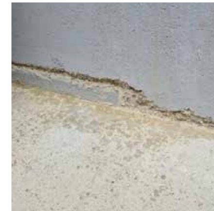
Mix the Teknocem HBR as per product instructions, and force into the gap with a gloved hand for initial contact coat, then build up flush with trowel.
