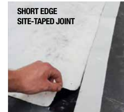
For detailing use CombiSeal Tape applied to the black side of the membrane ensuring a lap of 150mm.
