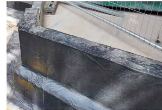
All right-angle internal corners should be smoothly filleted using Teknocem HBR to eliminate sharp transitions and reduce stress on the membrane, while careful attention should also be paid to corners, changes in direction, and exposed slab edges to ensure the detailing remains tidy and robust.
