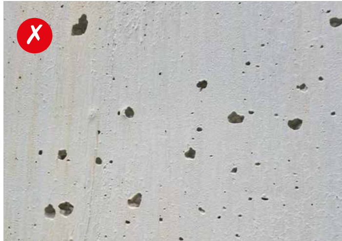
Surface prior to preparation. This substrate would not be suitable to receive a coating of Hydroseal FX.
