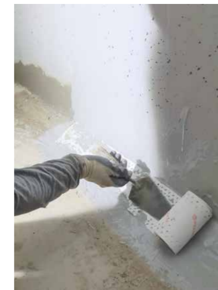
Hydroband 2000 is to be applied over any areas susceptible to cracking. Apply a 2mm layer of Hydroseal FX and embed the Hydroband 2000 into the layer. Then apply a second 1mm layer of Hydroseal FX over the top of the Hydroband 2000.
