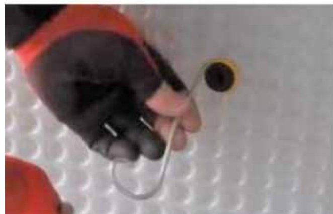
5mm diameter wall ties (Screw-in) can be used for brick/blockwork which are threaded into the pilot hole in the Hydroflow QS Plug.
