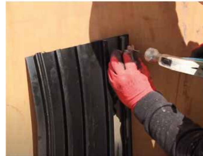
Hydrobar should only be fixed through the flanges onto a firm flat substrate such as a concrete.
