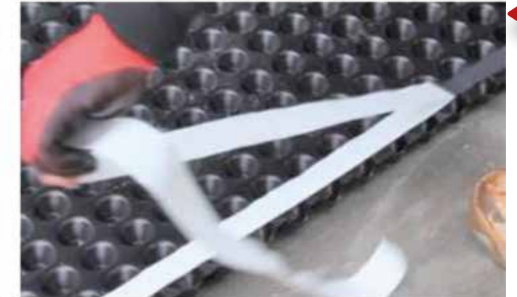
Remove release paper from Butyl tape.
