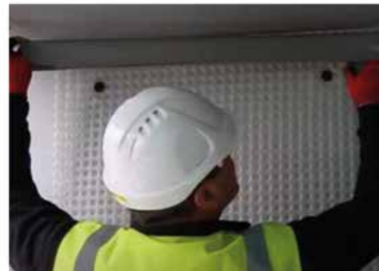
Using Hydroflow Corner Tape, seal the Hydroflow HP8 to the Hydroprufe Primer. Also overtape each membrane lap with Hydroflow Corner Tape.
