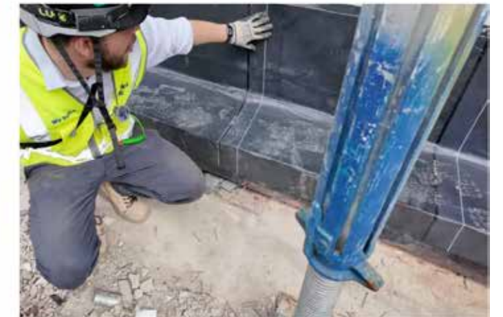
All right-angle internal corners should be smoothly filleted using Teknocem HBR to eliminate sharp transitions and reduce stress on the membrane, while careful attention should also be paid to corners, changes in direction, and exposed slab edges to ensure the detailing remains tidy and robust.
