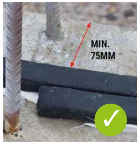
Joints in Hydrostop BR should be overlapped by a minimum of 50mm side-by-side. Install with a minimum of 75mm concrete cover to face of concrete.
