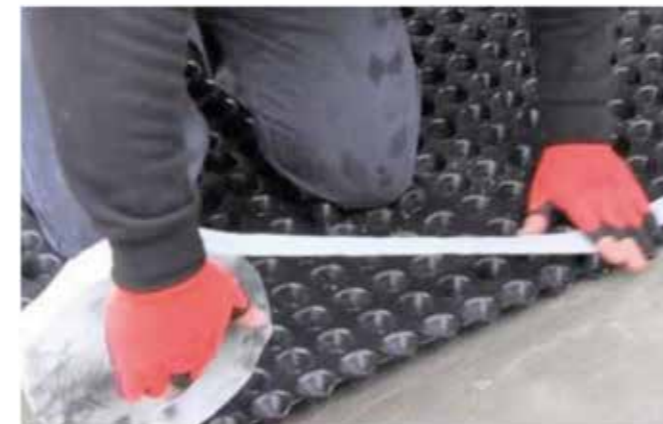
Apply strip of Hydroflow Butyl Tape to seal lap of Hydroflow HP20.
