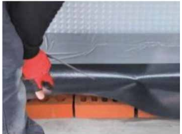
Where designed, install engineering bricks at the base of the wall and ensure the perp joints are left open.
