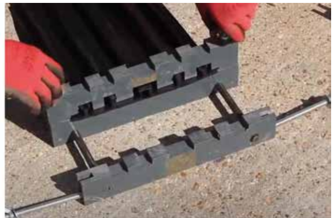
Tighten jig firmly leaving 10mm of the Hydrobar protruding.
