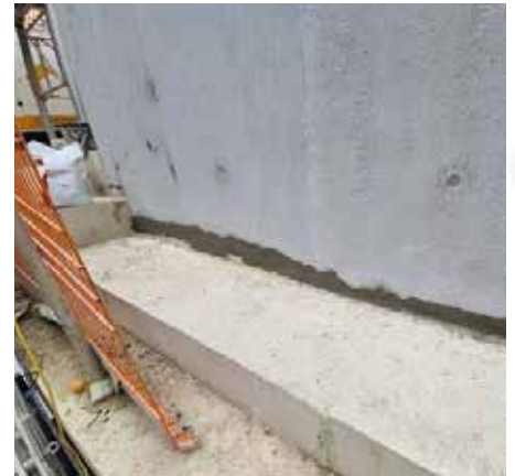
Mix the Teknocem HBR as per product instructions, and force into the gap with a gloved hand for initial contact coat, then build up flush with trowel.
