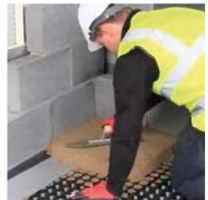
Once complete, Hydroflow HP20 is ready to receive floor screed.
