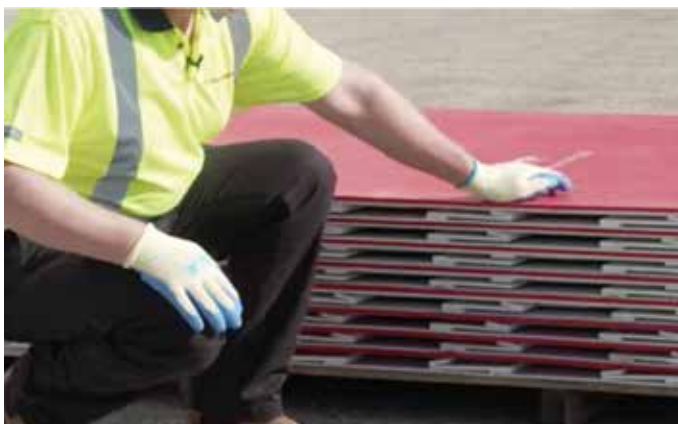
Place the Void-Tek flat panels near to installation area.
