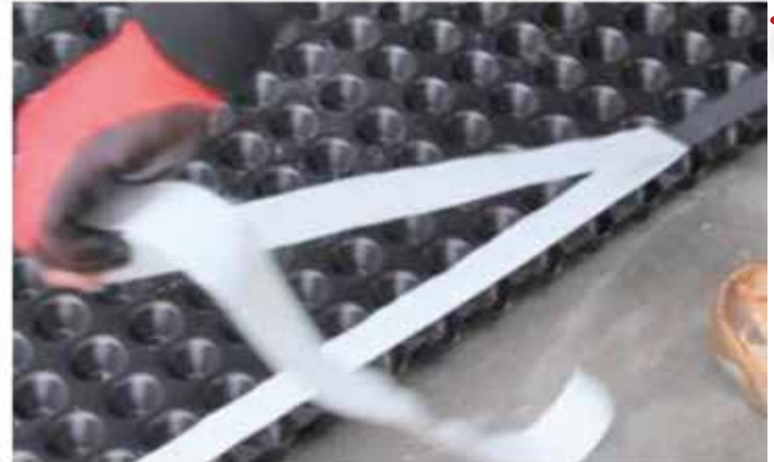
Remove release paper from Butyl tape.
