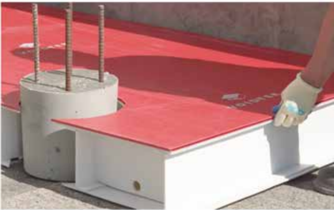
Place in position, lowering over the pile.
