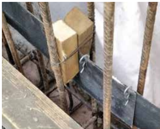
Cemflex VB should be pre-installed in kicker joint before concrete is cast. This can be hung with tying wire and timber blocks as pictured above, or Omega Holders can be supplied.
