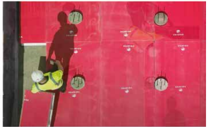
Continue to place all Void-Tek panels to cover the required area.
