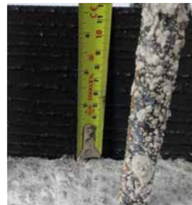
Ensure waterbar is installed with 30mm embedment into first pour, leaving 120mm protruding for wall pour.
