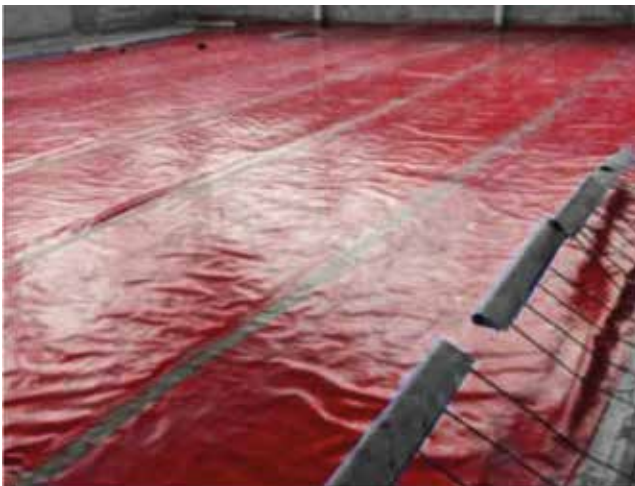
Membrane prior to protection board installation.
