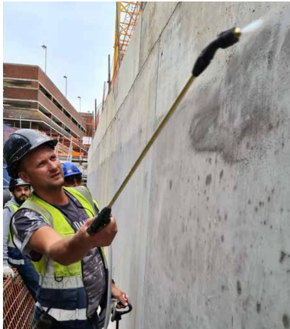
Surface prior to preparation. This substrate would not be suitable to receive a coating of Hydroseal FX.
