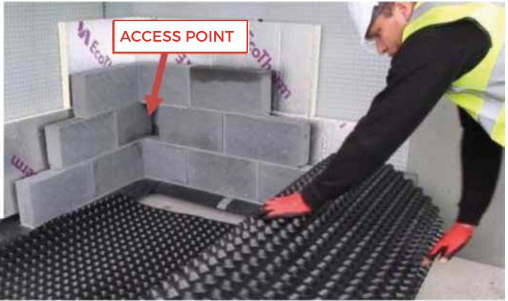
Roll Hydroflow HP20 out on the floor with studs facing down.
