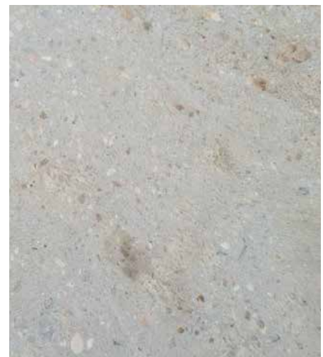
Example of correctly prepared substrate.
