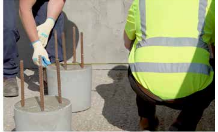
Accurately measure the pile cap diameter.
