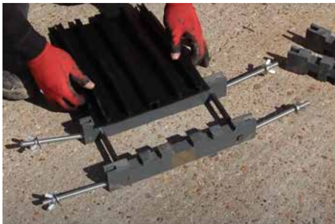
Lay Hydrobar onto the jointing jig.
