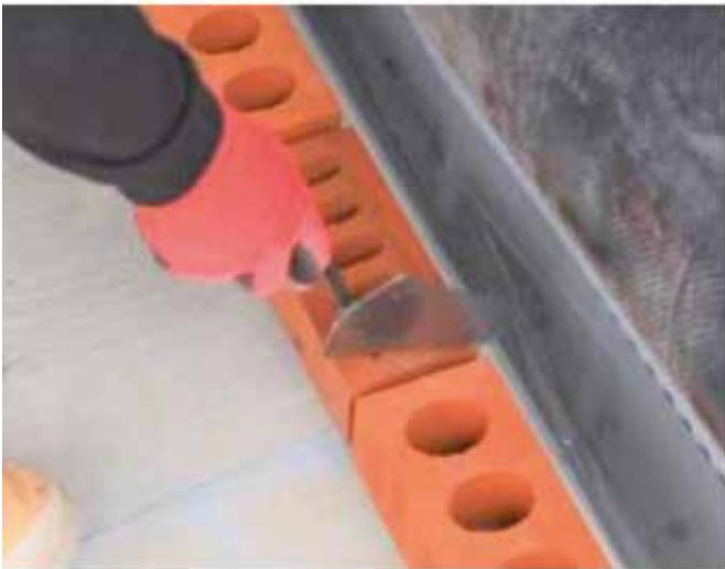
Where designed, install engineering bricks at the base of the wall and ensure the perp joints are left open.
