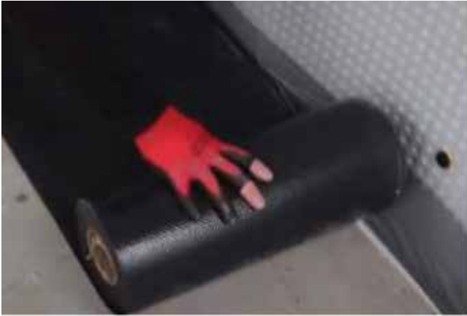
Roll out Hydroprufe DPC and seal to the Hydroflow HP8 using Hydroflow Corner Tape around 300mm above the floor.
