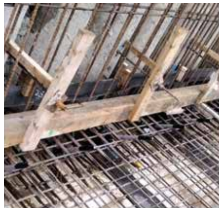
Cemflex VB to be secured between starter bars.
