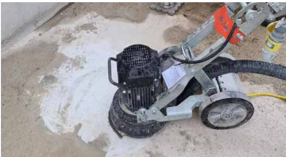
To prepare the horizontal areas, a diamond grinder or powerful jetwasher should be used.
