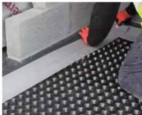
Tape the Hydroprufe DPC to the Hydroflow HP20 using Hydroflow Corner Tape.
