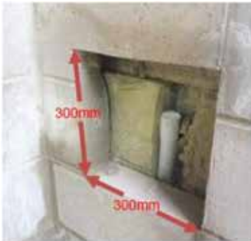
Recommended minimum access hatch size.
