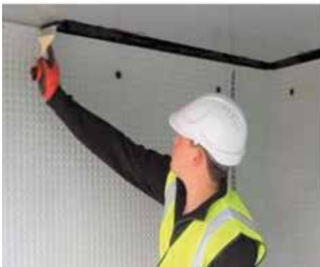
Apply 150mm Strip of Hydroprufe Primer to soffit. Leave to cure.
