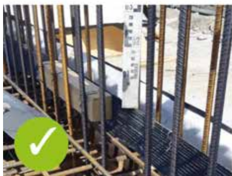
Laser level used to ensure correct consistent height.
