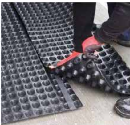
Ensure that Hydroflow HP20 is overlapped by a minimum of two studs and pushed firmly down to ensure the lap is sealed.
