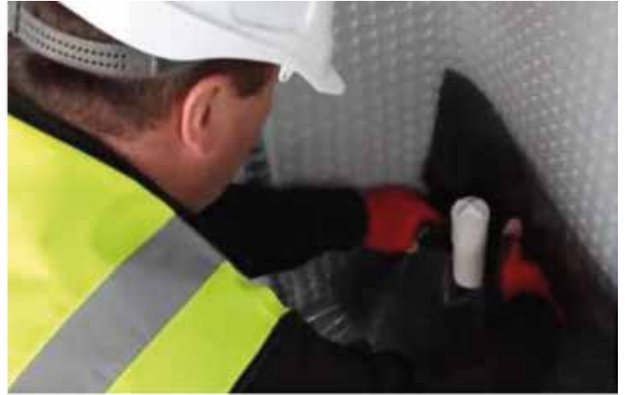
Cut a small perforation for the flushing point pipe and tape to the Hydroprufe DPC. Ensure DPC is firmly taped to the Hydroflow HP8.
